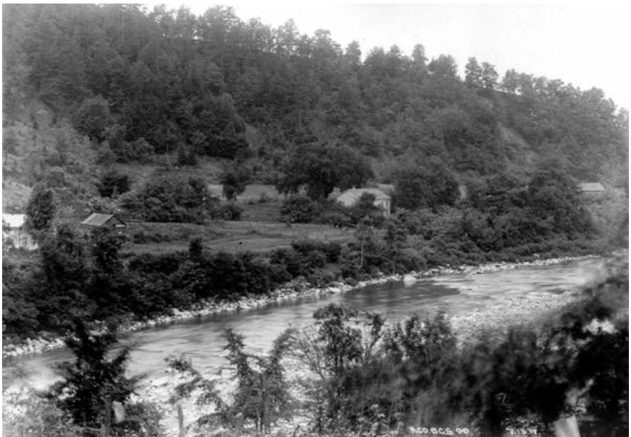
The remaining cotton mill structures. Courtesy of the Gilboa Historical Society
