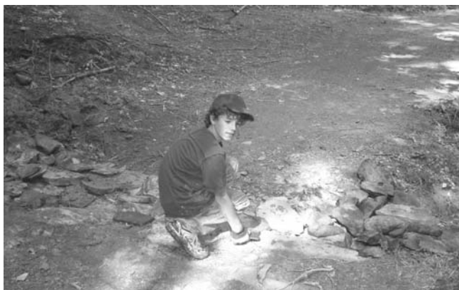
Owen Nied of the Schoharie County Youth Bureau and the Cobleskill-Richmondville School working on a water diversion on the Minekill Falls Trail.
