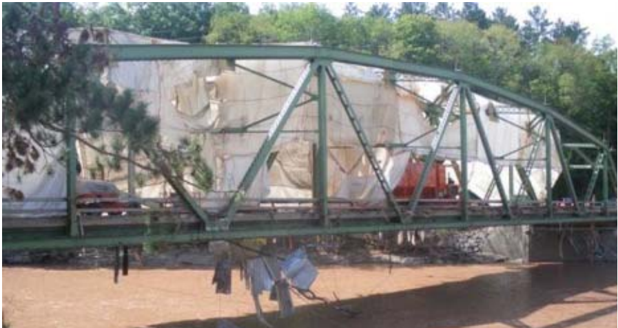
The Prattsville bridge, September 1, 2011. The plastic sheeting is used to contain the sandblasting materials within the construction site, and the bridge was reopened 6 months later by the Department of Transportation, March 19, 2012. This picture copyright © Albany Times Union . 9/2/12, used with permission, courtesy of the Albany Times Union .
