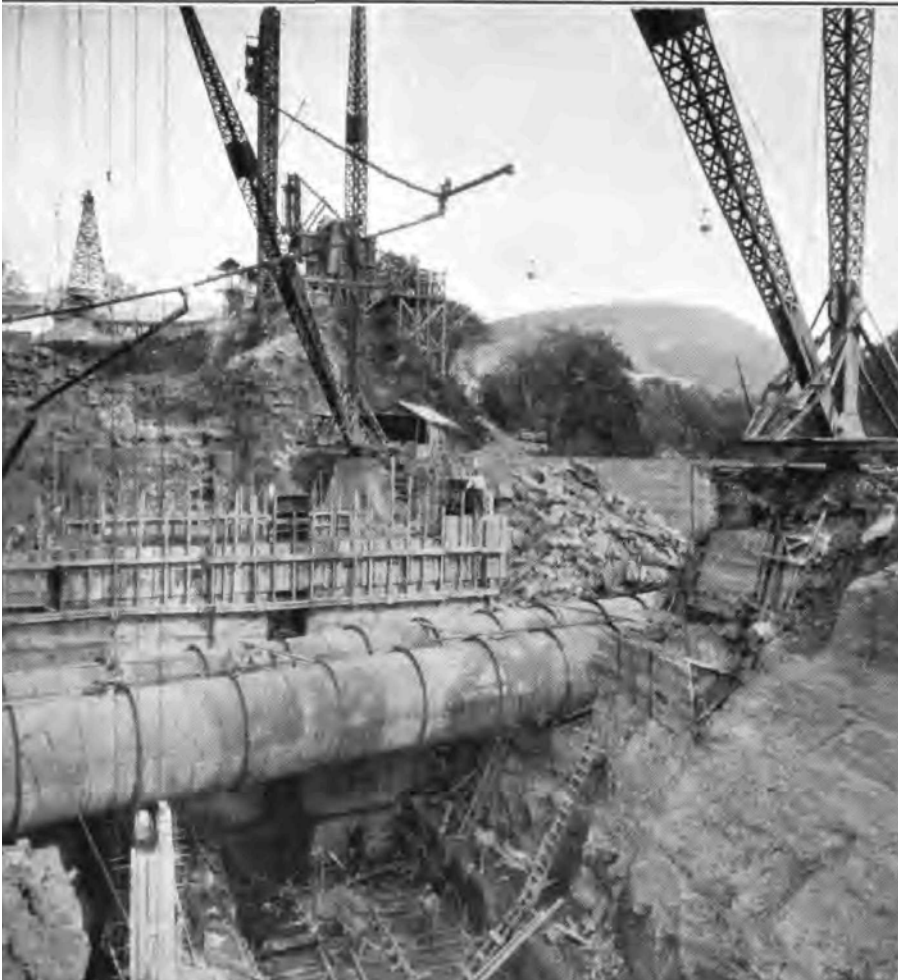
The 2 large steel pipes were integrated into the work site as it evolved in the years to come. Here, the pipes were routed right through the foundation excavation. Board of Water Supply Annual Report 1921, photo courtesy of Department of Environmental Protection.
