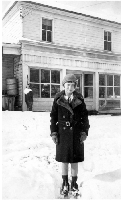
My older sister, Geraldine, outside the Mackey General Store, ca. late 1930s. Note the newly installed electric service at the top left corner of the building.
