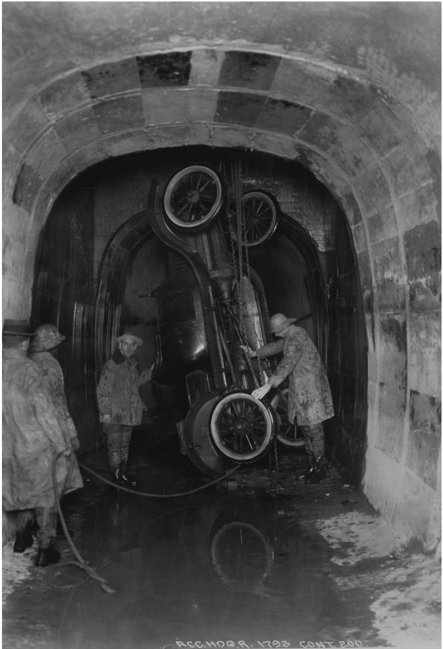
At Shaft 5, the cars were hoisted on end, pivoted, and their direction reversed. January 6, 1924, courtesy of the Department of Environmental Protection.
