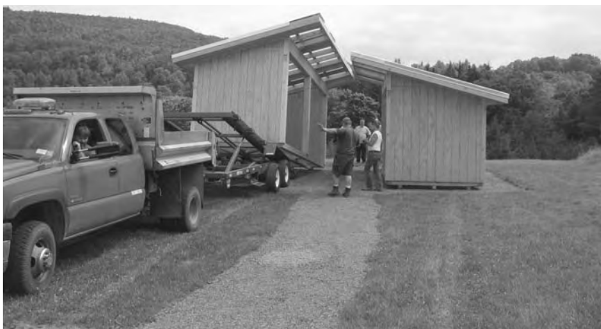
Dennis Muthig and his robotic truck placing the second half of the barn.
